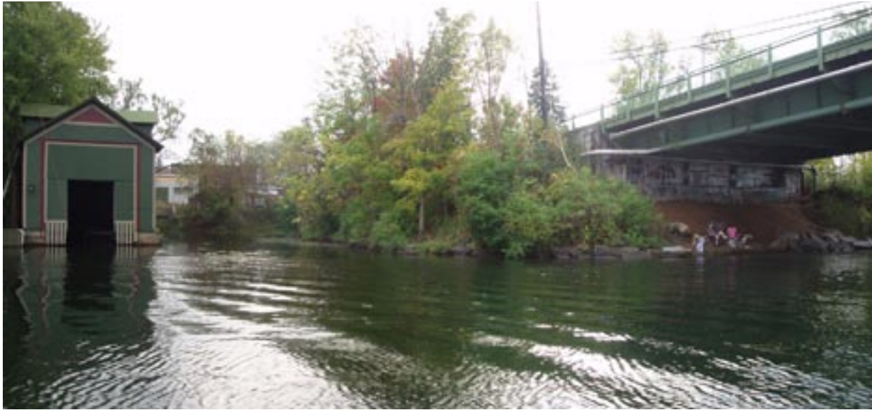
Existing view of Route 11 Bridge abutment
