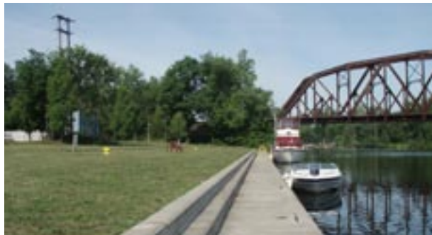
View west in Riverfront Park. Visitors coming by car or boat underutilize this park. Improved vehicle and pedestrian access, additional amenities, and better organization would attract more visitors to this park and make it a vital public destination.
